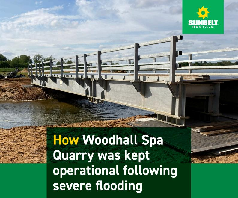
Access was restricted to Woodhall Spa Quarry following severe flooding in the Lincolnshire area. A temporary bridge was created to allow vehicular access in the area affected, keeping the quarry operational.
